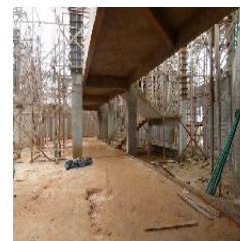
Vista do Bloco A, ala central
